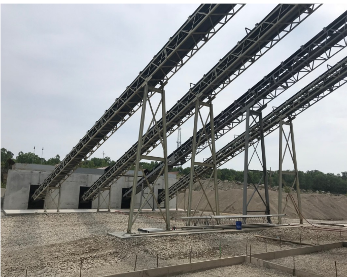
Four aggregate conveyers from the ground hoppers to the overhead aggregate bins in the plant. Precast wall panels manufactured and erected by ALD Precast.
