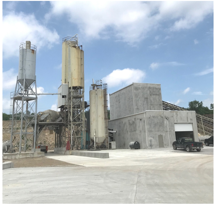
Newest silo for slag cement on the left
