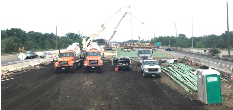
The Ruhlin Company I-71 over 270 north of Stringtown Road 660 yard bridge deck
