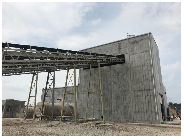
Four aggregate conveyers from the ground hoppers to the overhead aggregate bins in the plant. Precast wall panels manufactured and erected by ALD Precast.
