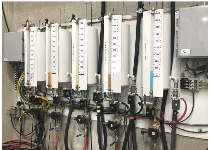
New Sika admixture dispensing system
