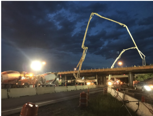
Above and right: Barrier Wall on I-71 with Shelly & Sands, Spring/Summer 2019
