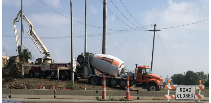
Shelly & Sands pouring a bridge footer at I-71/Frank Road
